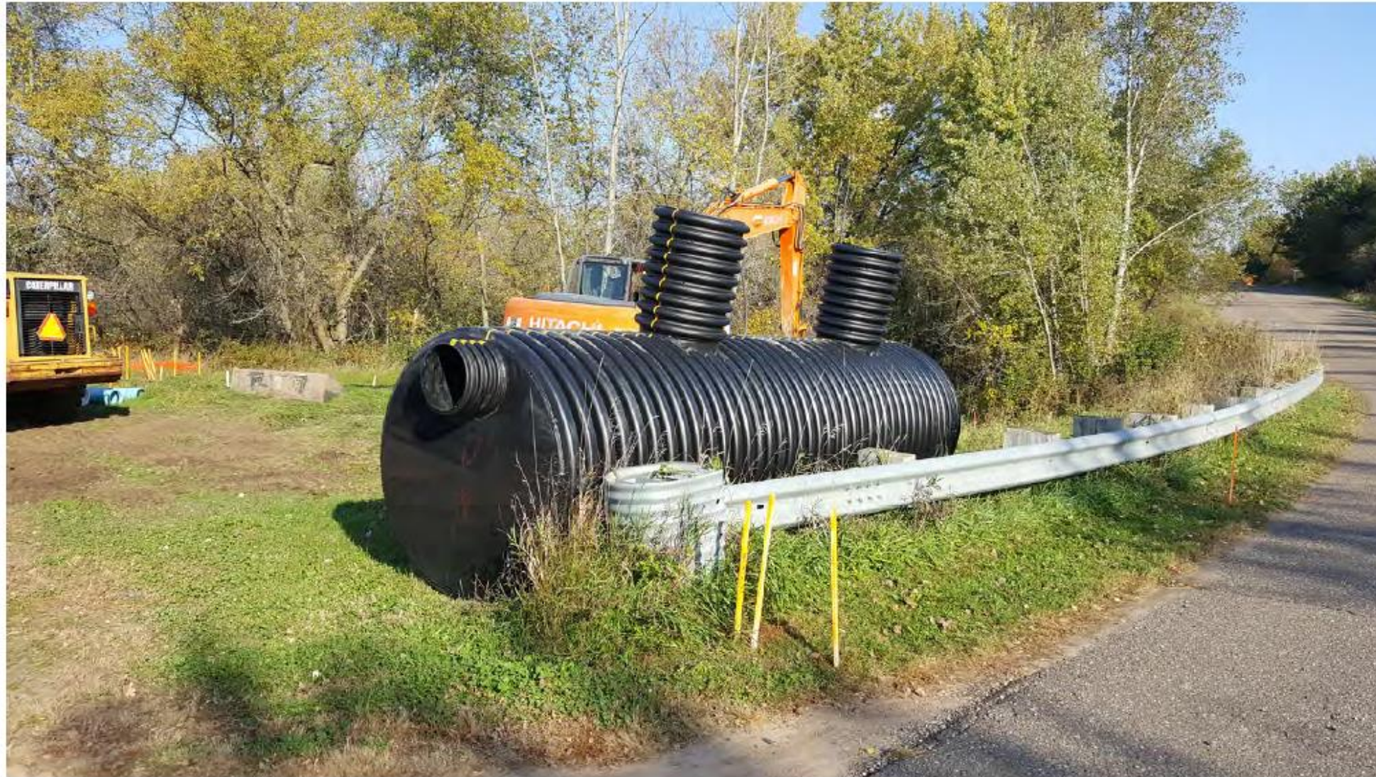
Stormwater Quality Tank Pre-Installation (EOR)
