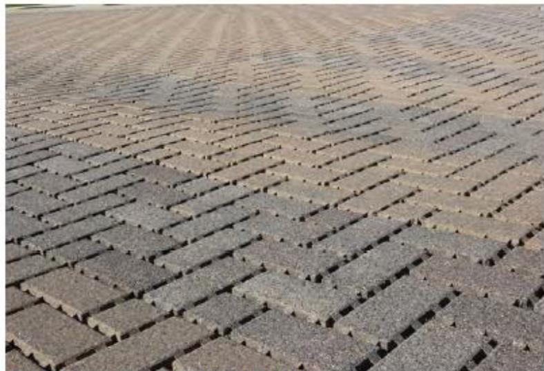
Permeable Pavers, installed (EOR)
