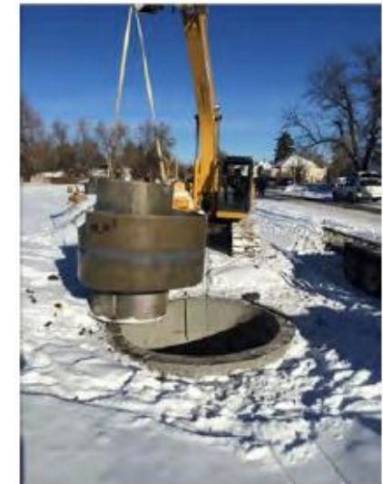
Hydrodynamic Separator (CDS Stormwater Treatment)
