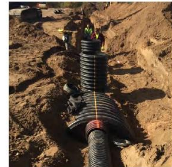
Embedded Stormwater Quality Tank (Prinsco)
